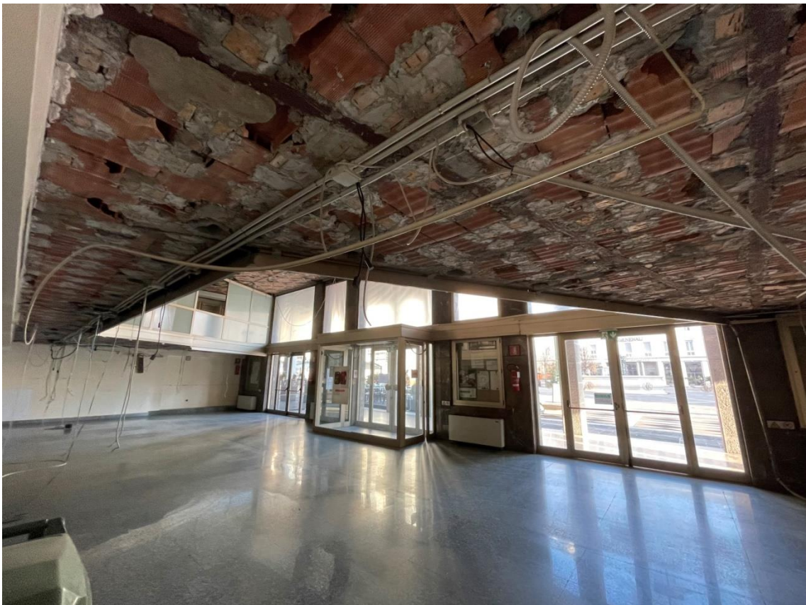
Vista piano terra
