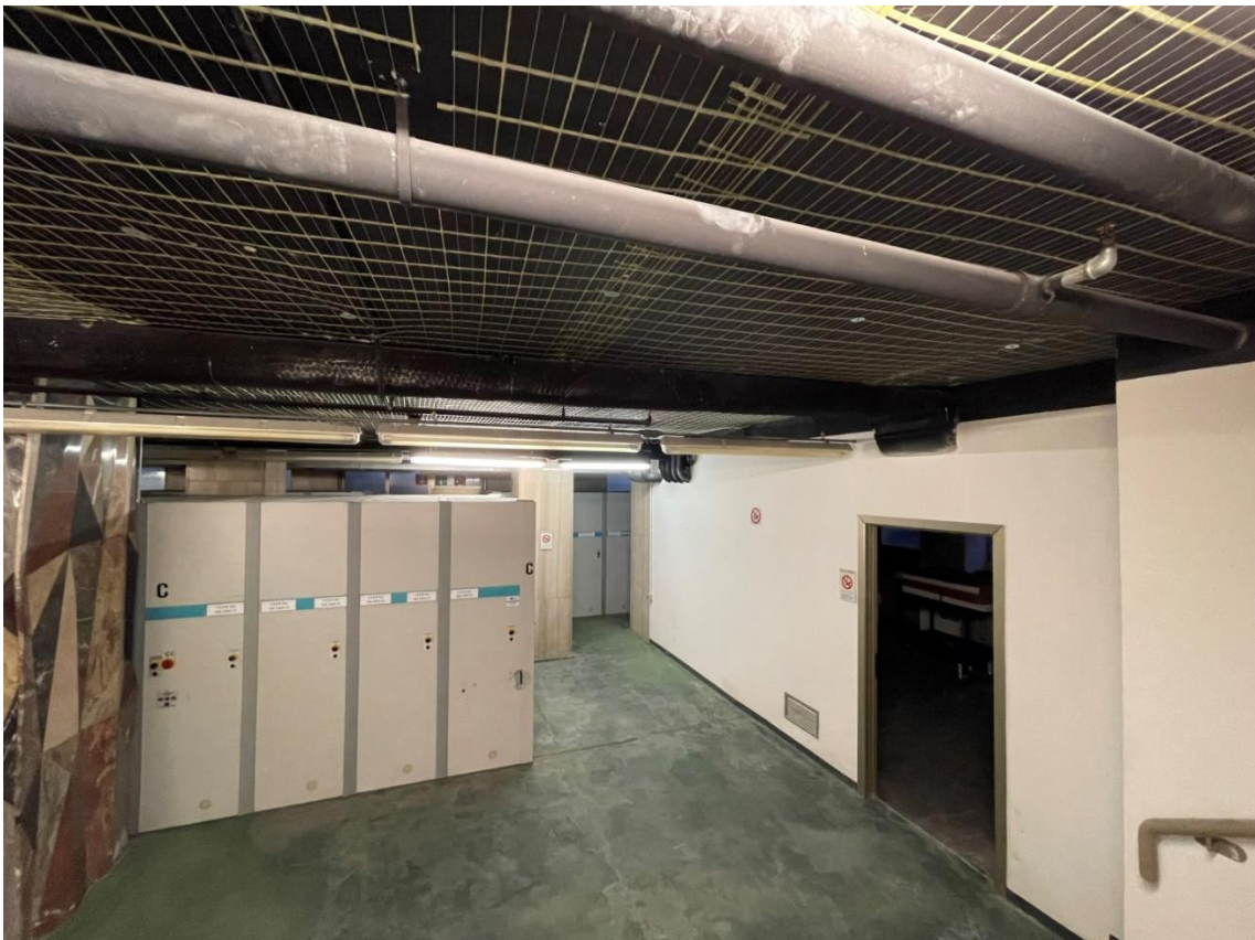
Vista piano interrato
