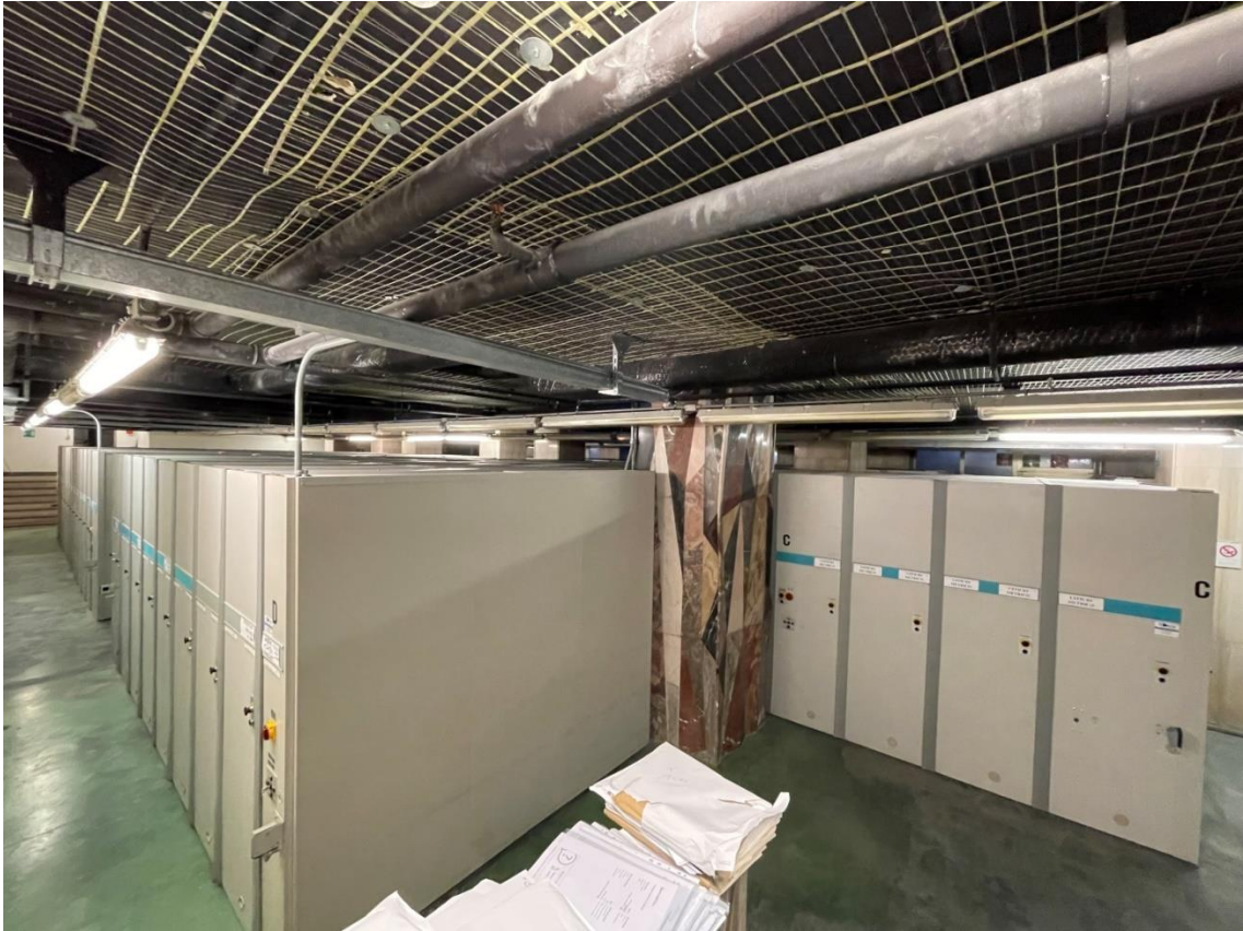
Vista piano interrato
