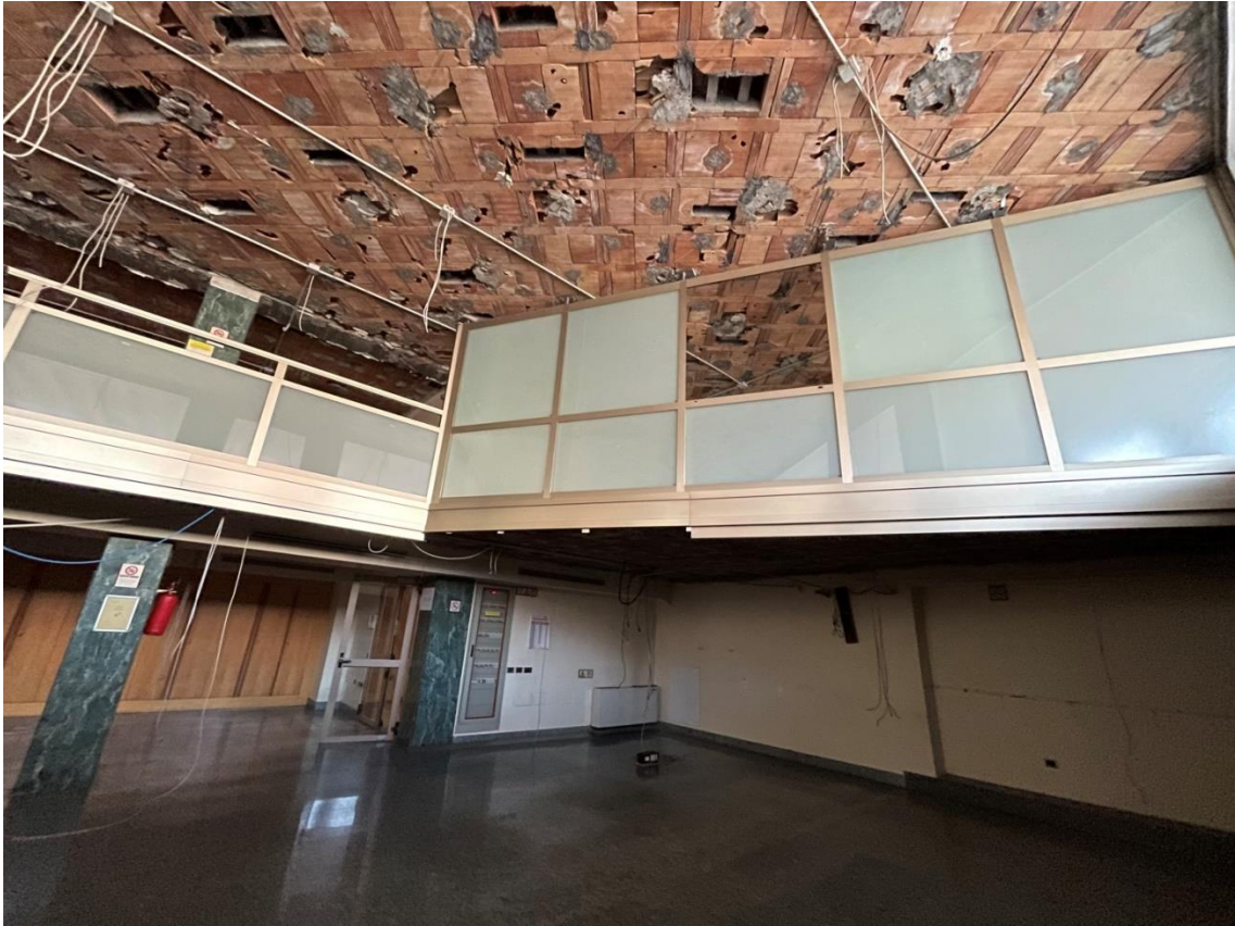
Vista piano terra
