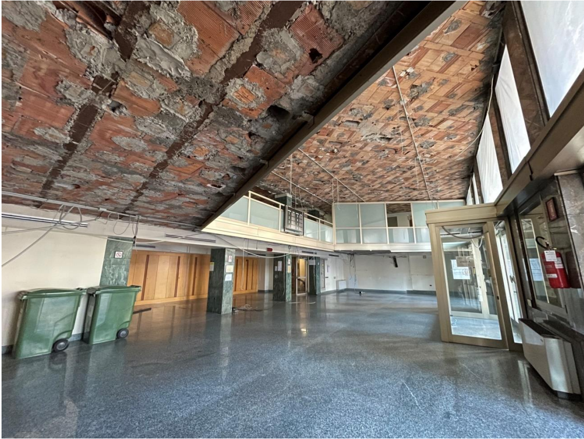
Vista piano terra
